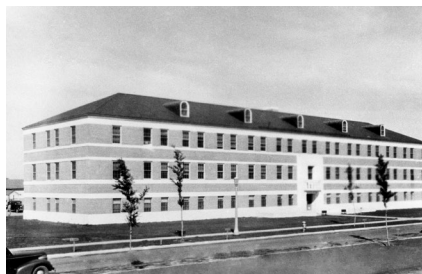
Barracks and Post Exchange, Hill Field, 1941.
